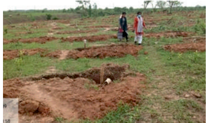
Mulching and Plantation around SMC structure
